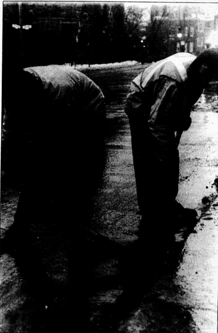
City workers Bruno Raymond, left, and Ronald Bray, work during driving rain Tuesday to clear drains of ice and slush so the water will run off properly.
