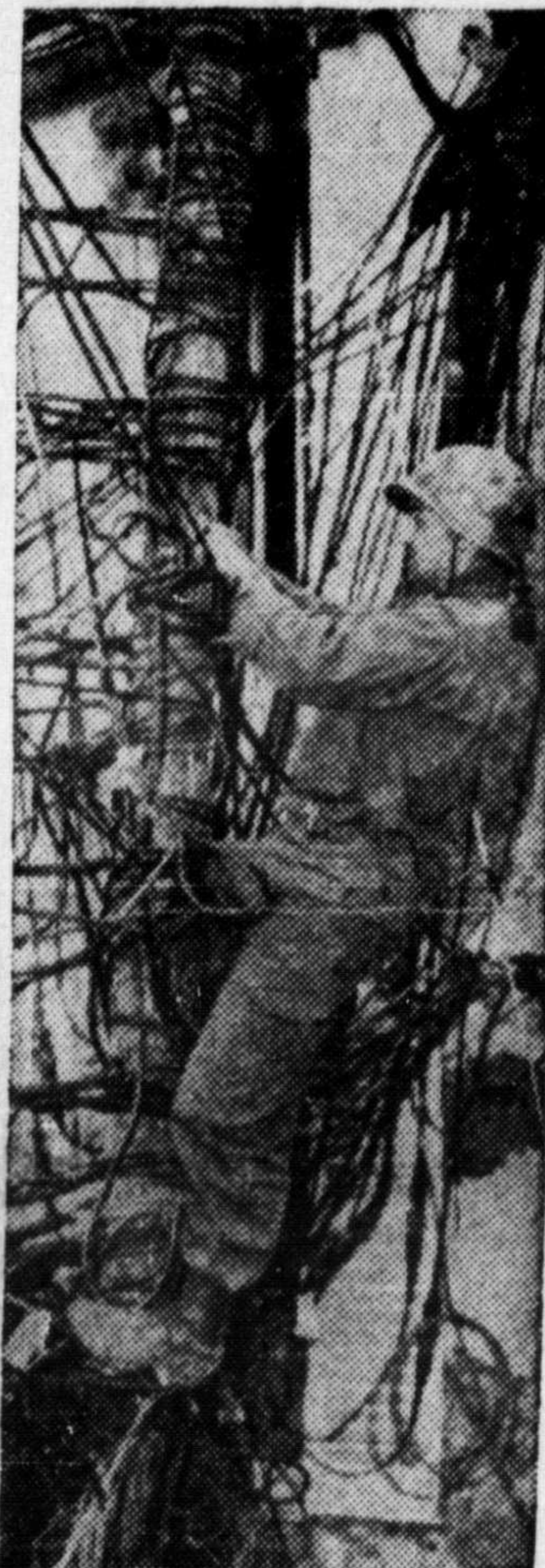
Installing a switchboard system for U. S. First Army headquarters in Normandy, a sergeant gets to work on tangled maze of wire outside switchboard room.
