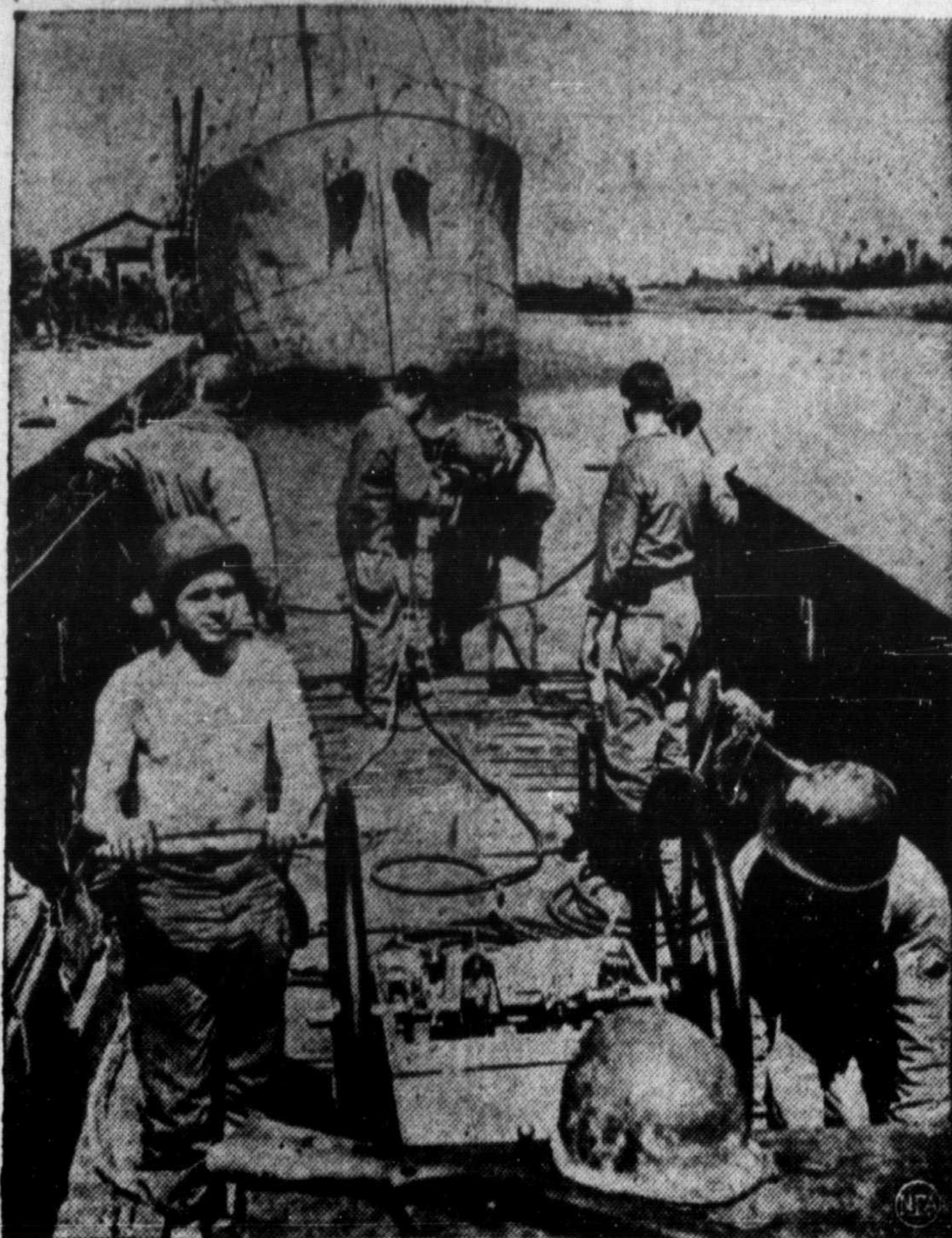
U. S. Army diving unit, believed to be the only one in France, is kept busy clearing rivers and canals of mines and underwater obstructions. Unit works from an LCVP (landing craft, vehicle and personnel). In background, diver's tender helps diver don his helmet before going down to inspect canal bed a few miles behind front.
