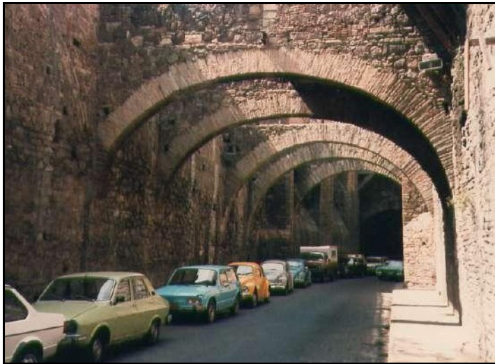
Figure 10.9: Underground tunnel with a parking space.
