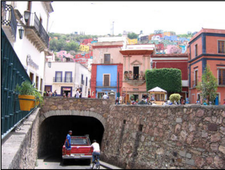
Figure 10.8: Entrance to a tunnel.
