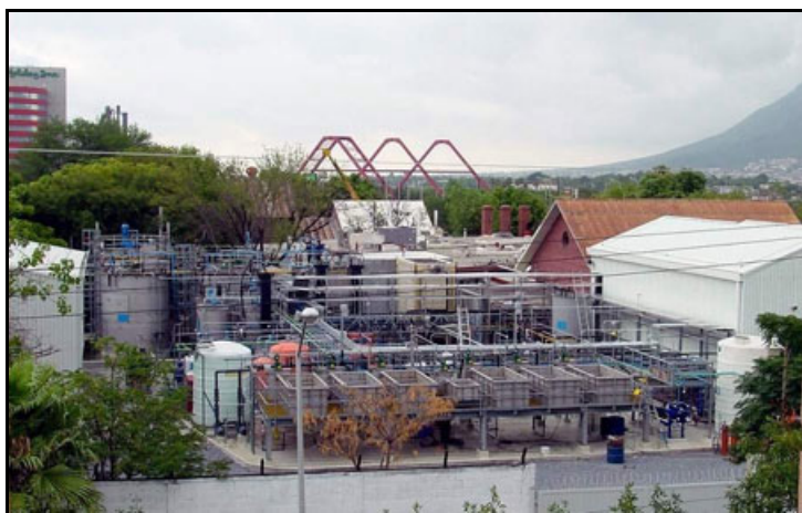
Figure 6.1: Peñoles chalcocopyrite bacterial leaching pilot plant.
