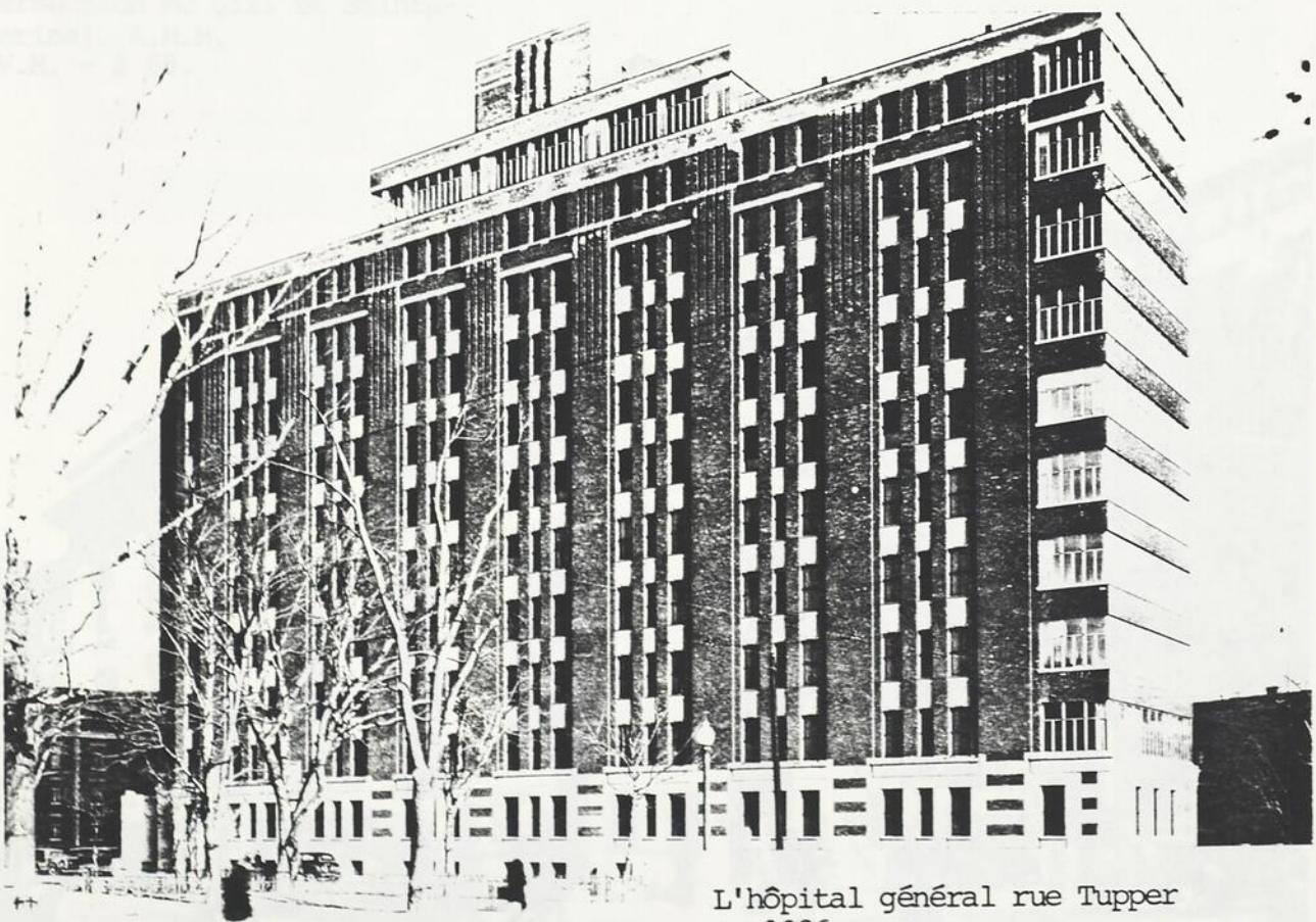
Montreal General Hospital A.M.M. S.U.V.M. - 34099.
