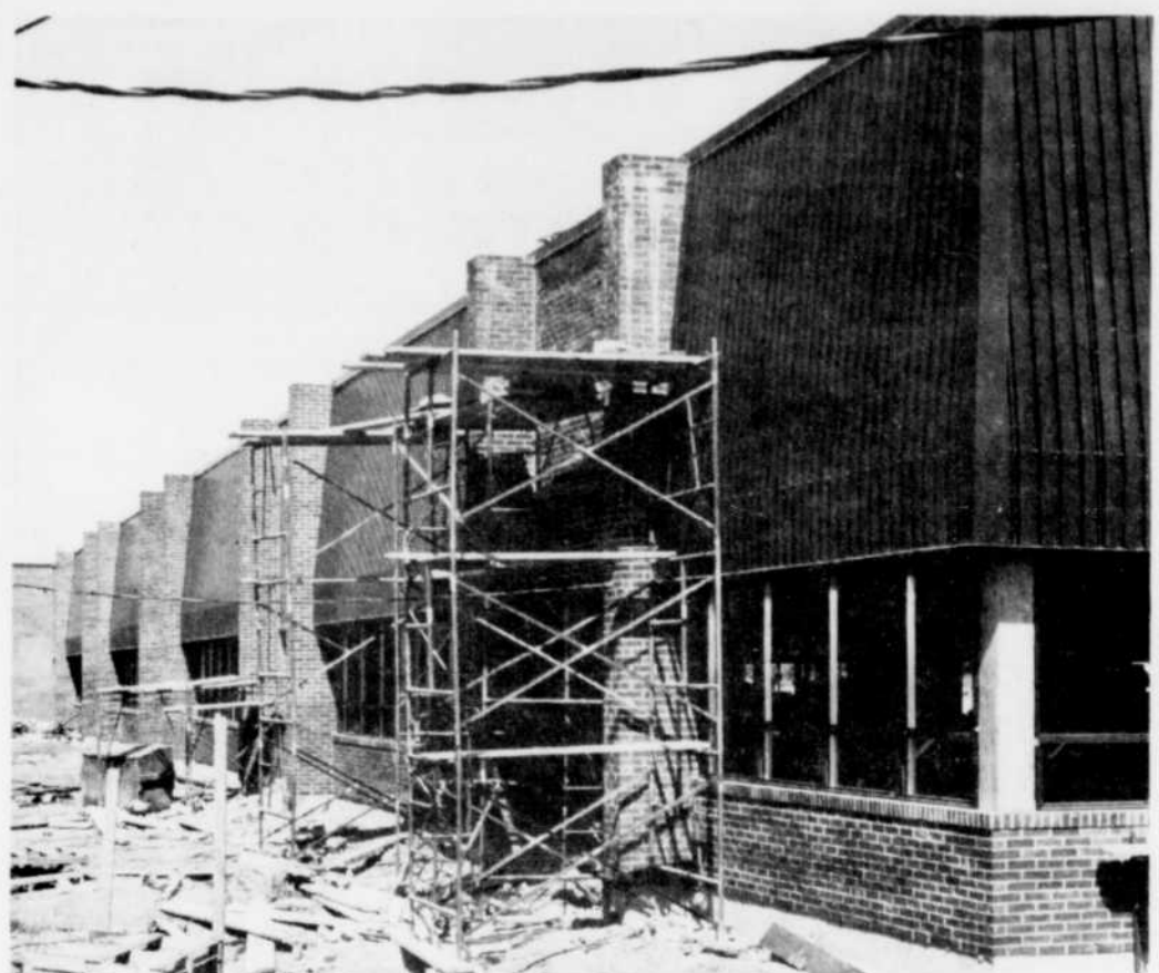
THE SNOWDON CAMPUS OF VANIER COLLEGE UNDER CONSTRUCTION DURING THE MONTH OF JULY ON DECARIE BLVD. NEAR QUEEN MARY ROAD.
