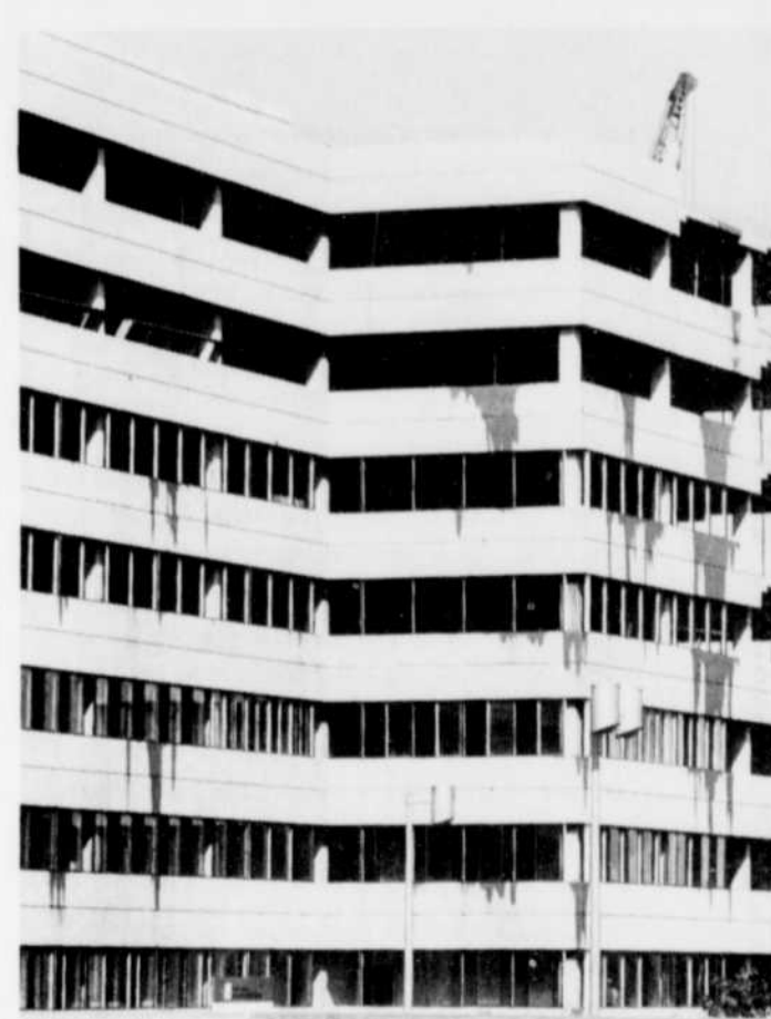
JOHN ABBOTT COLLEGE'S KIRKLAND CAMPUS UNDER CONSTRUCTION IN MID-JULY.
