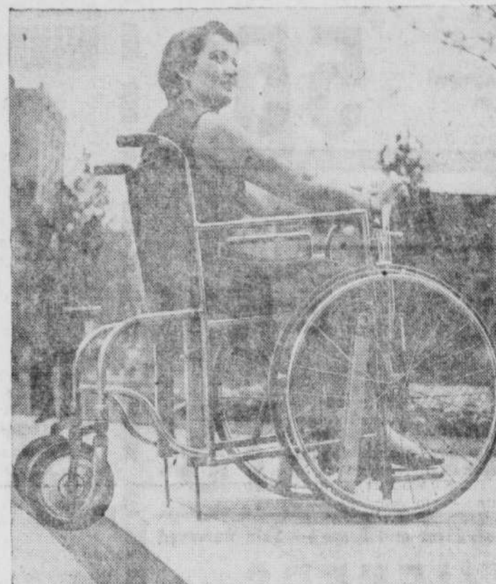
Front steel legs retracted, she uses rear leg action to finish climb. Jamie is paralyzed from the waist down.
