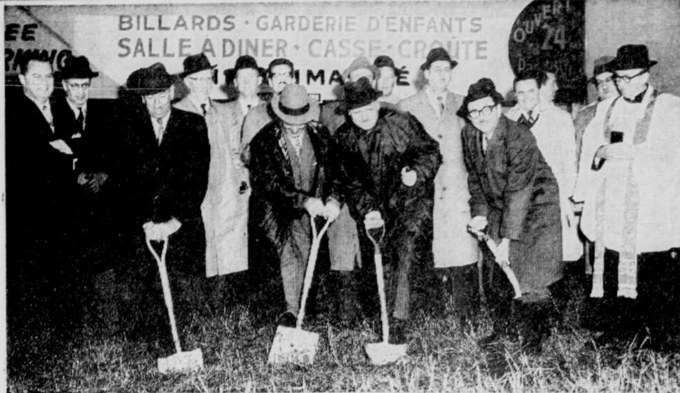
SOD TURNED — Three mayors and a member of parliament are seen in the act of turning sod where the Normandie Lanes, a new 48-lane bowling layout, will be built. Left to right, Mayor S. Blais of Bromptonville, Mayor J. W. Bernier of Rock Forest, Mayor Armand Nadeau and Maurice Allard, MPP, form the shovelling brigade. In the rear are some of the invited guests who attended the special ceremony. On the right is Rev. Father Valere Duplain parish priest of Rock Forest, while on the left is Guy Ouenneville, manager of the proposition. The new building will be built on Bourque Boulevard just beyond the Alouette Motel in Rock Forest.
