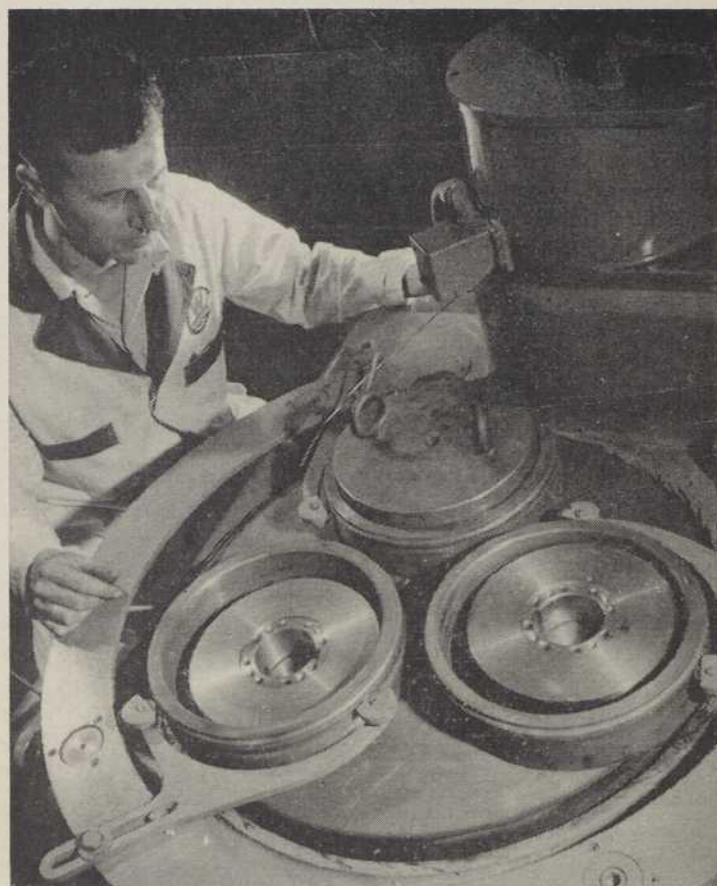
SUPER-FINISHING ON SPECIAL GRINDING AND LAPPING TOOL.
