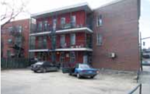
📍 The landscaping project at the Habitations Lenoir-Saint-Antoine.
