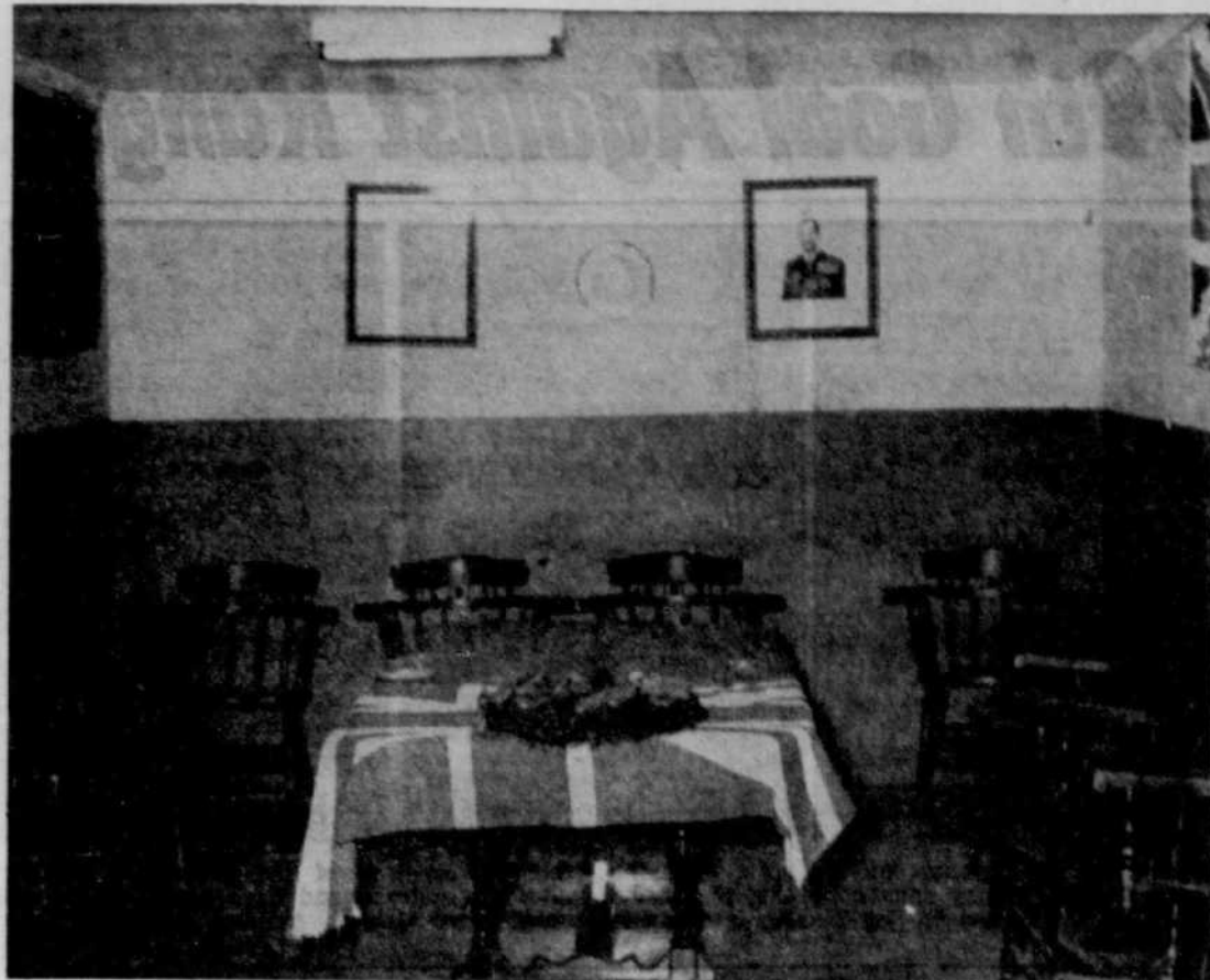
Veterans' Hall Annex — The committee room of the newly-completed Army, Navy and Air Force Veterans' Association Hall annex on Main St. is shown above. Entirely built by the members, the annex also houses a new refreshment counter and a furnace room.
