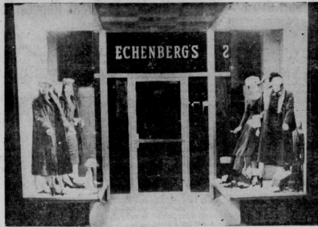
Echenberg Store Renovations — Above is shown the new show windows and entrance of Jack Echenberg and Sons store, Wellington street north, which has undergone extensive renovations recently.
