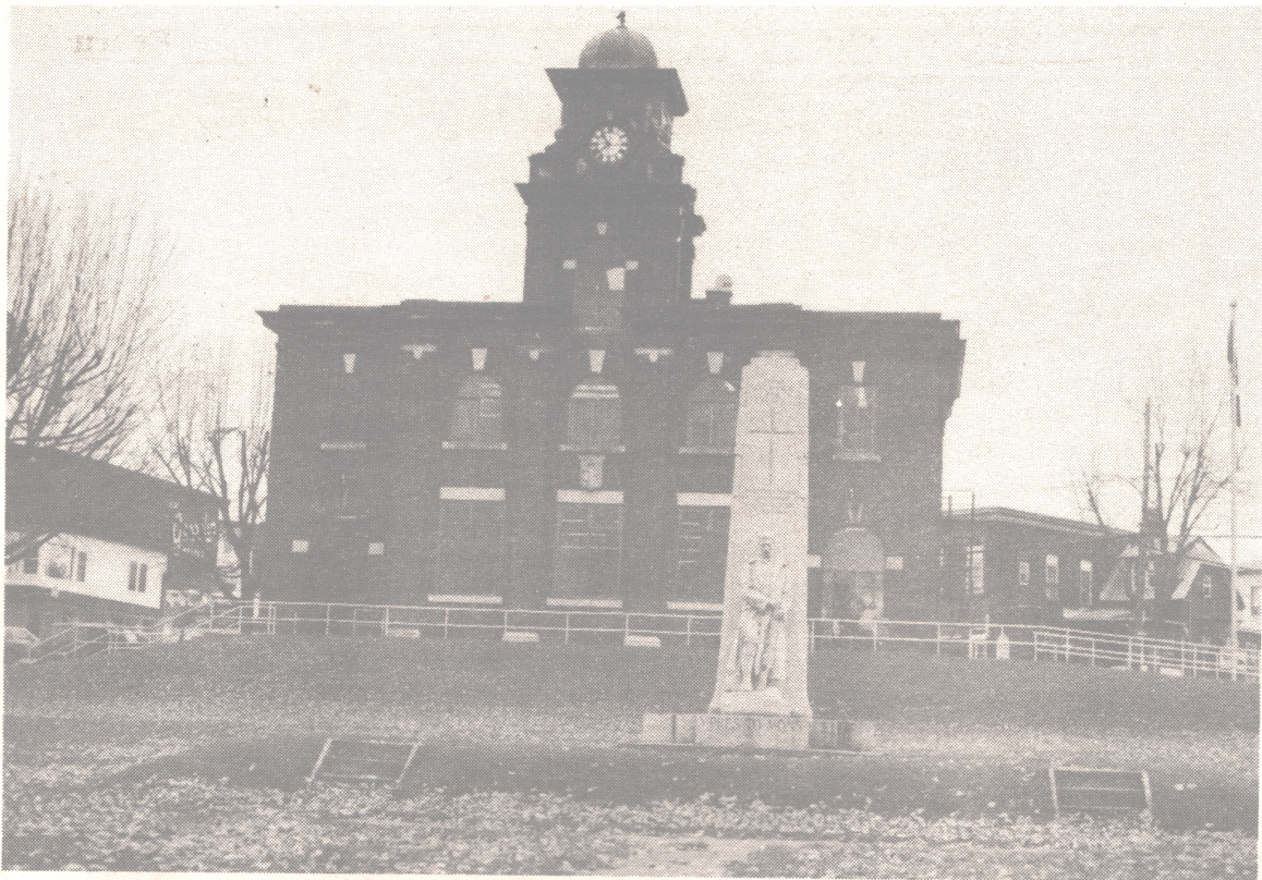
The beautiful Post Office building also houses Employment Canada
