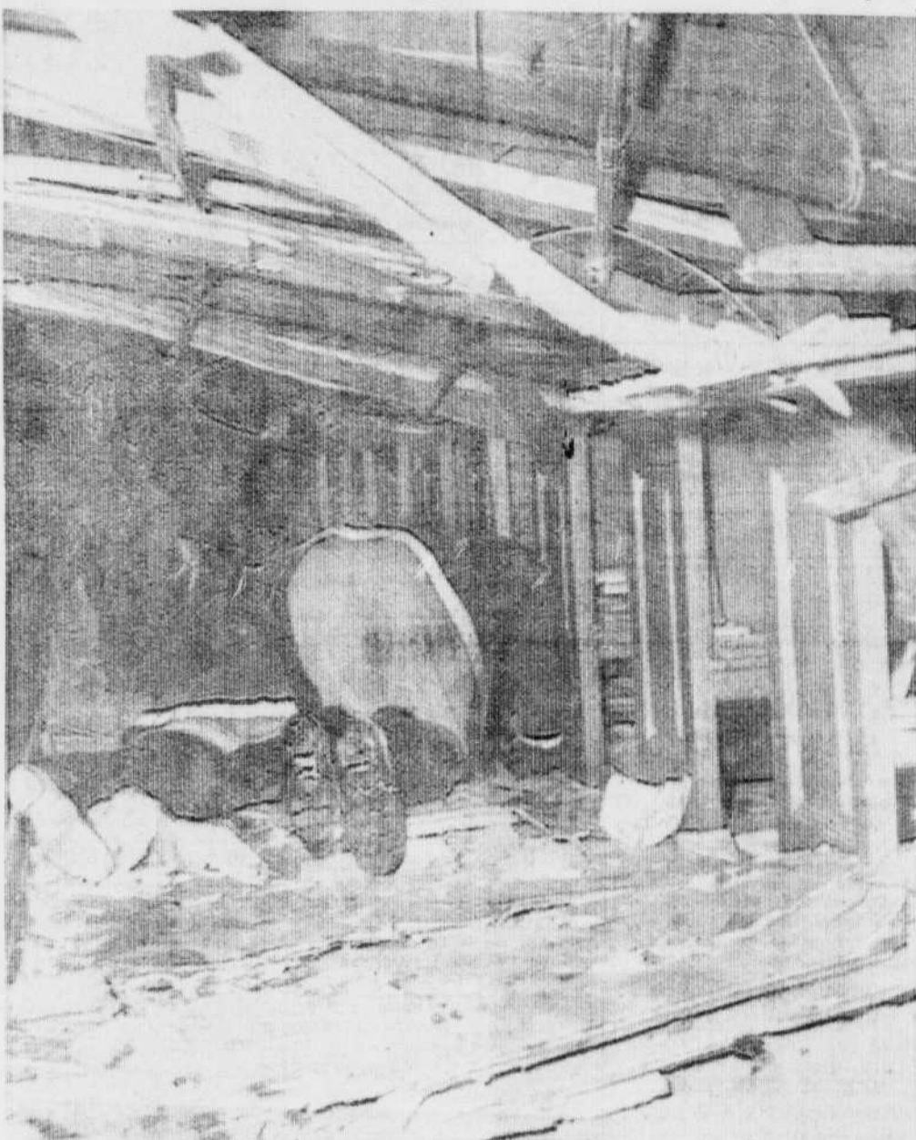
SEARCHING FOR VICTIMS — Firemen crawl along the pews of the St. Rose of Lima Church, Baltimore, Md. looking for injured after the roof collapsed. Wreckage of the roof is resting on the sturdy oak pews, which saved the lives of many. Forty-six were treated in hospital. (AP Wirephotos)
