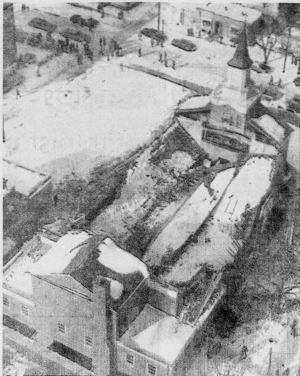
ROOF COLLAPSES — The roof of St. Rose of Lima Roman Catholic Church, Baltimore, Md. collapsed during 8 o'clock Mass yesterday. The roof collapsed following a snowfall of about 11 inches earlier this week. (AP Wirephoto)
