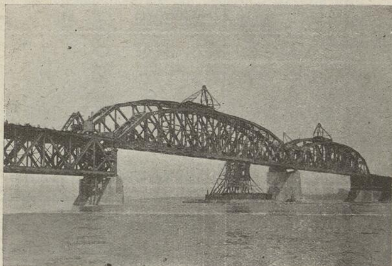
Bridge over the St. Lawrence River at Lachine, P. Q.
