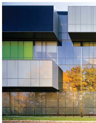
CCIT COMMUNICATION, CULTURE AND INFORMATION TECHNOLOGY BUILDING UNIVERSITY OF TORONTO AT MISSISSAUGA SAUCIER + PERROTTE ARCHITECTES PHOTOGRAPHE MARC CRAMER
