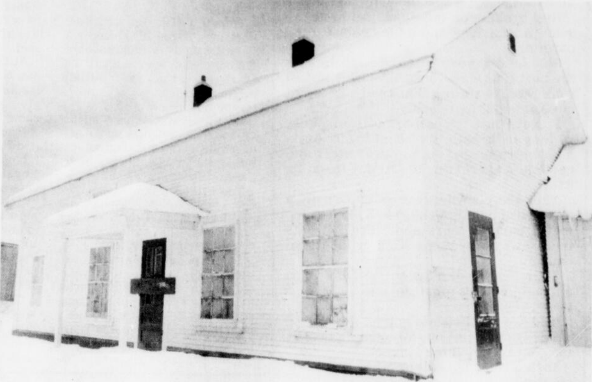
The decomposing bodies were found in this house on Route 143.
