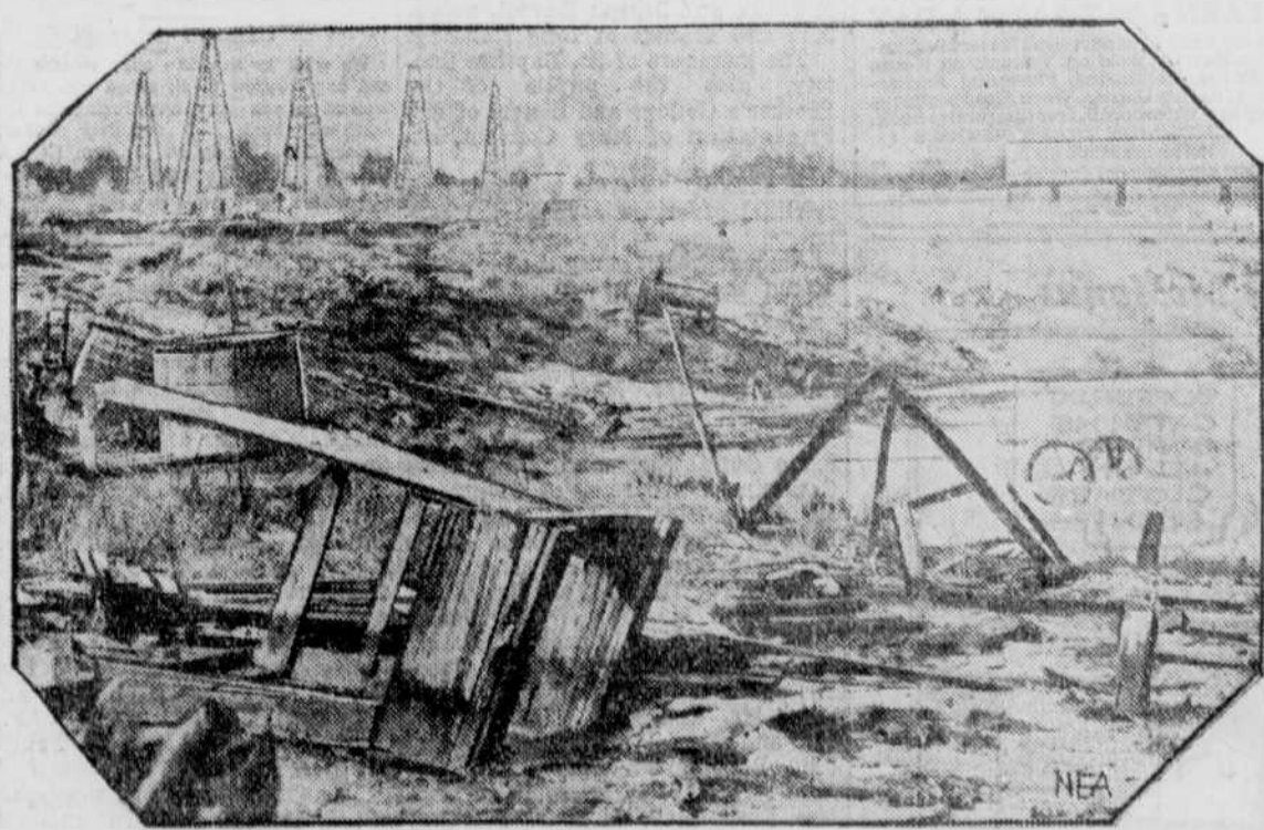
Here's a bird's-eye view of where 10 acres of land in the Sour Lake, Texas, oil field sank without warning burying derricks, tool sheds and other structures in a crater 100 feet deep. The queer prank of nature caused some nearby flowing wells to stop producing, while others increased their output. The power house at right, was wrecked a short time after this picture was taken.
