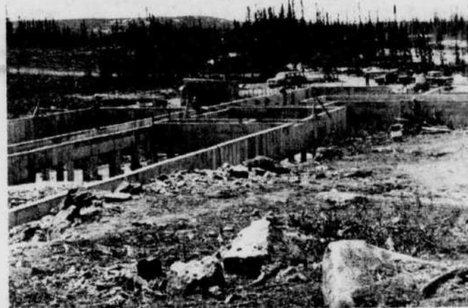
NEW TOWN STARTING UP — Building foundations are laid on the site of a permanent town being constructed at Churchill Falls, in central Labrador. A temporary community near the Churchill Falls power project now holds more than 1,500 people. The new town's population is expected to reach as high as 7,000 at the peak of the power project. (CP Photo)
