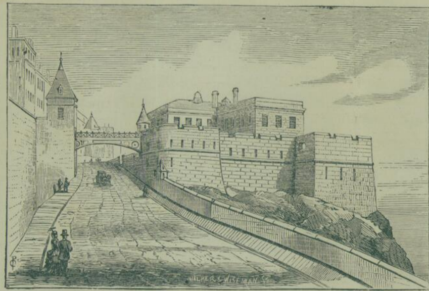
MOUNTAIN HILL.—Iron Bridge.
