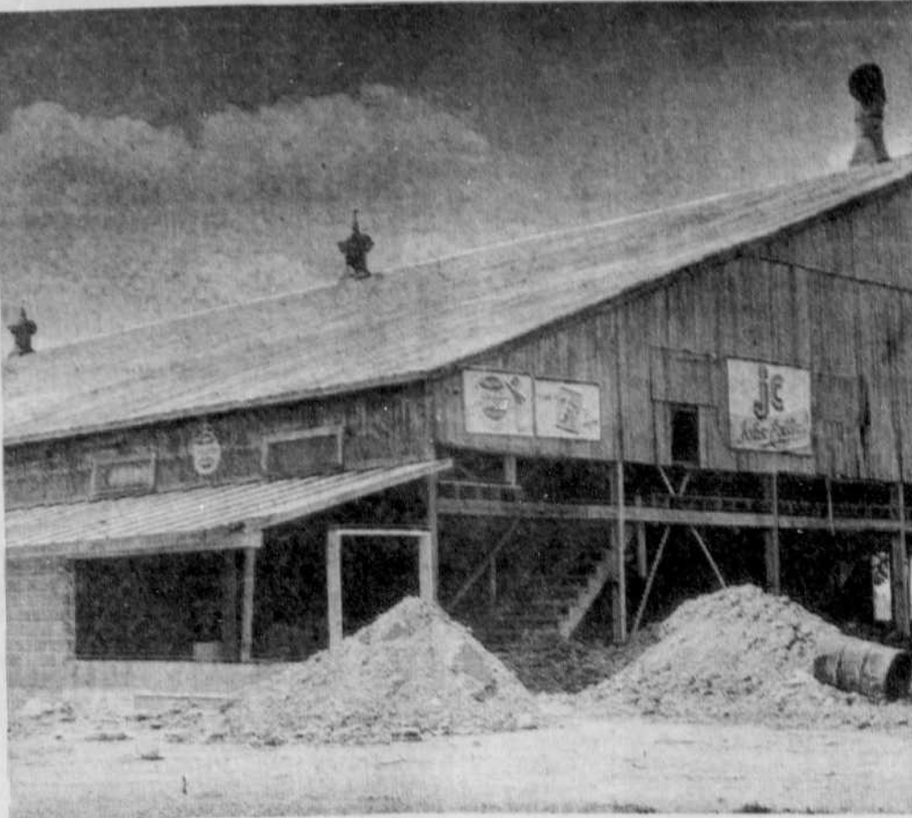
ARENA REPAIRS — Waterloo's arena begins to show improvement as work starts on renovating the old building. Town council voted $3,000 for improvements to the building. (Record photo by Harvey Mitchell)
