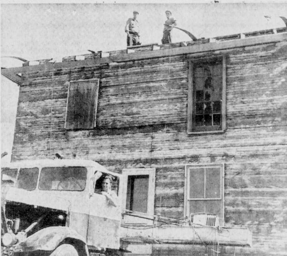
OLD HOME MOVED — A float carries a two-storey Waterloo home from Lewis Street to a new location just outside the town limits. The
