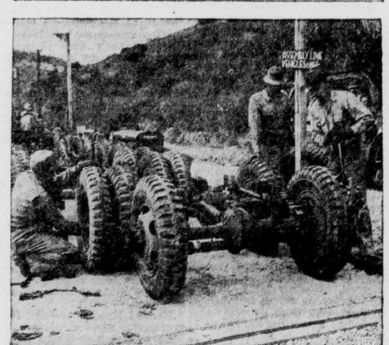
Mass production comes to the Southwest Pacific as American Army mechanics put war machines together in assembly line fashion at a base "somewhere down under." Here a truck that was shipped in sections is assembled in rush order time, while a row of heavy tires await the rest of the vehicles they'll roll.
