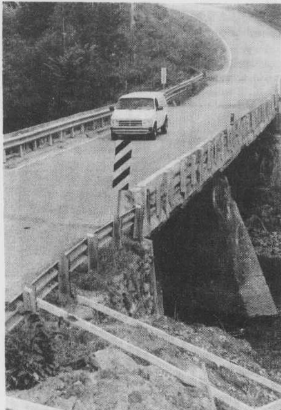
The old bridge has a centre pylon sitting on the river bed. The new structure will replace this with steel cables.
