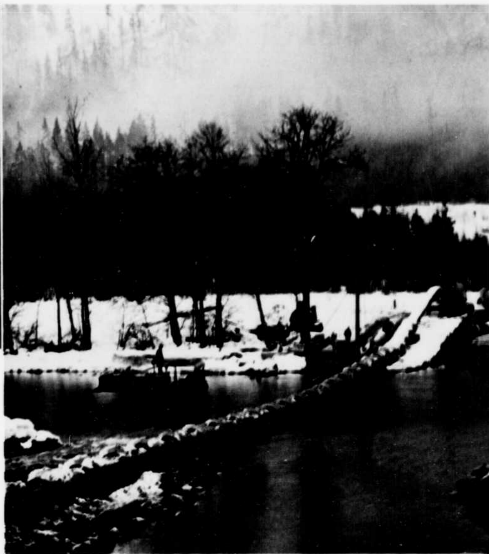
Construction du pipe-line West Coast Transmission, 1956.
