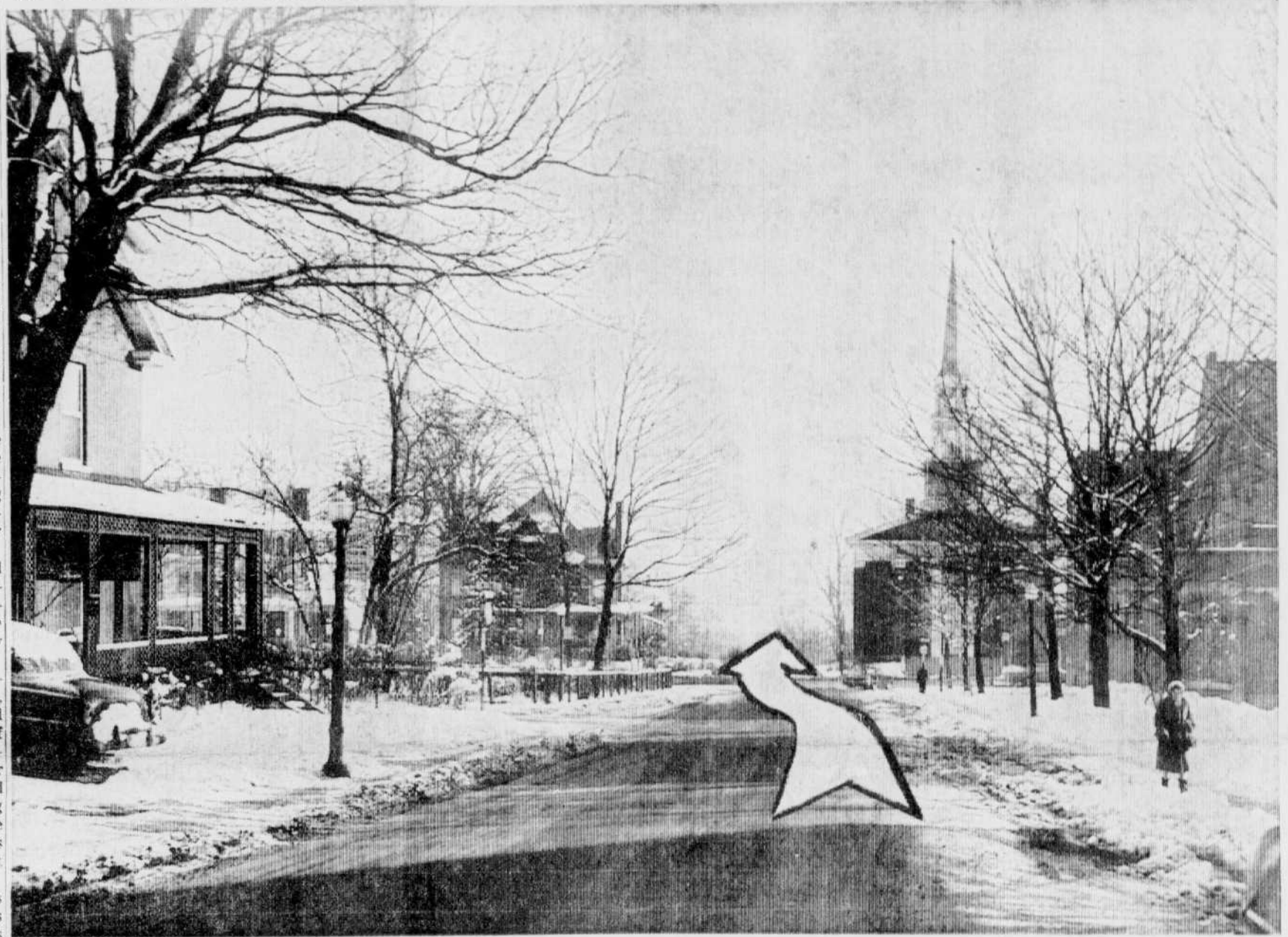
BRIDGE APPROACH — Above is the approach site to the proposed Montreal Street - Terrill Street bridge looking down Montreal Street towards the St. Francis River. Arrow shows how approach will have to be bent around the corner of Plymouth Church (background of picture). On the right is St. Peter's Church, and in the foreground, left, is the McKeage Rest Home. Immediately behind the rest home is Mitchell Park, around which it is proposed to construct a traffic circle.
