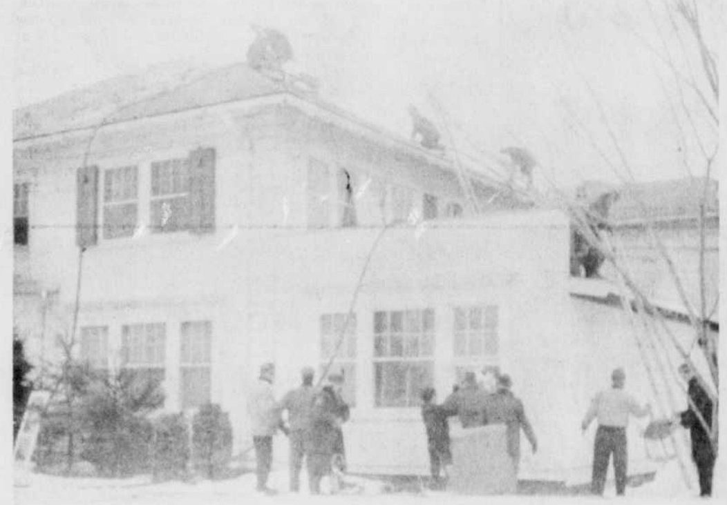
$100,000 DAMAGE — Men of two fire departments pour water between the walls in an attempt to douse flames at the
