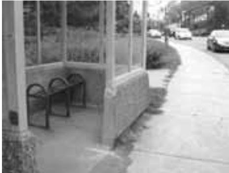
Northeast corner of Lansdowne.
