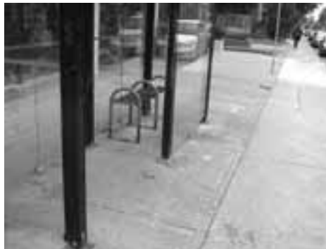
Southwest corner of Metcalfe.
