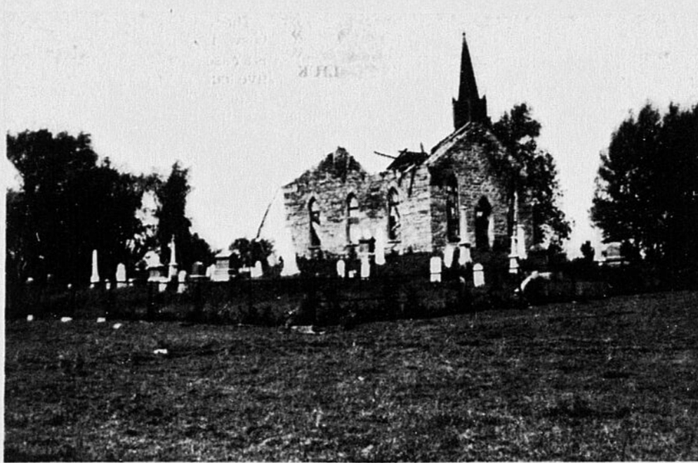
"Crumbling into ruins"
