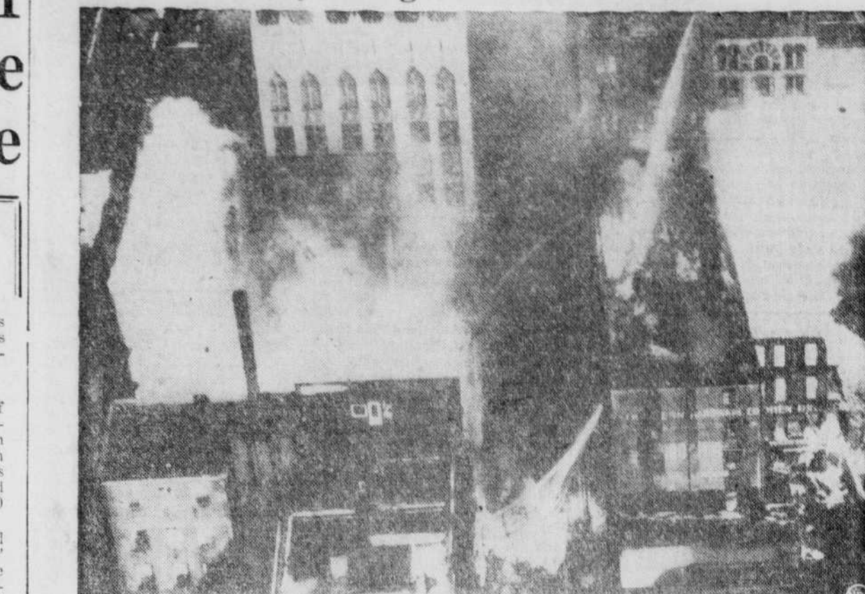
Air view of fire in Charleston, W.Va., which was fanned by strong wind and destroyed an entire block of warehouses, office buildings and stores. Blaze spread to one of city's largest hotels, driving its patrons into streets. Fire departments from communities outside Charleston were called in to help battle blaze in freezing weather. Damage to buildings alone totals $1,000,000, and no estimate was put on their contents.
