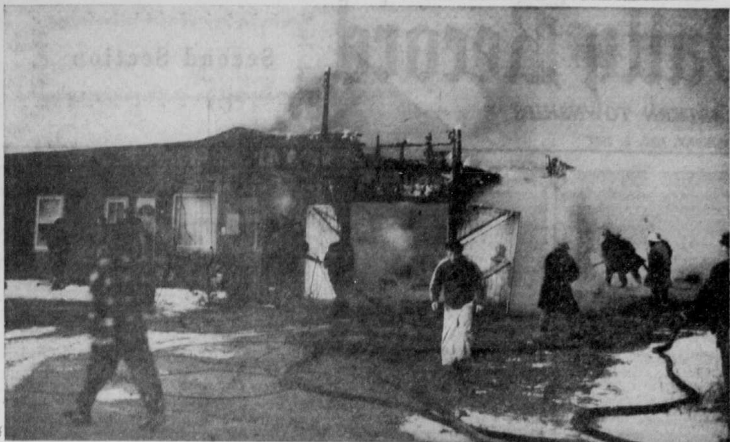
RESIDENCE DESTROYED --- Fire destroyed the home of Mr. and Mrs. Marcel Racicot, Yamaska Blvd., Sweetsburg, last week. Mr. and Mrs. Racicot and their four children were saved. The fire is believed to have started from a lighted oil-soaked rag being used to thaw pipes. (Record Photo by Gillespie).
