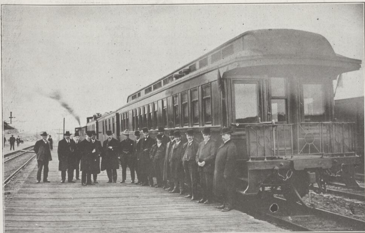
OPENING OF A NEW CANADIAN RAILWAY—The first train over the Toronto-Sudbury line of the Canadian Pacific Railway, and the officials of the road. (Photo by Gillespie, Sudbury.)
