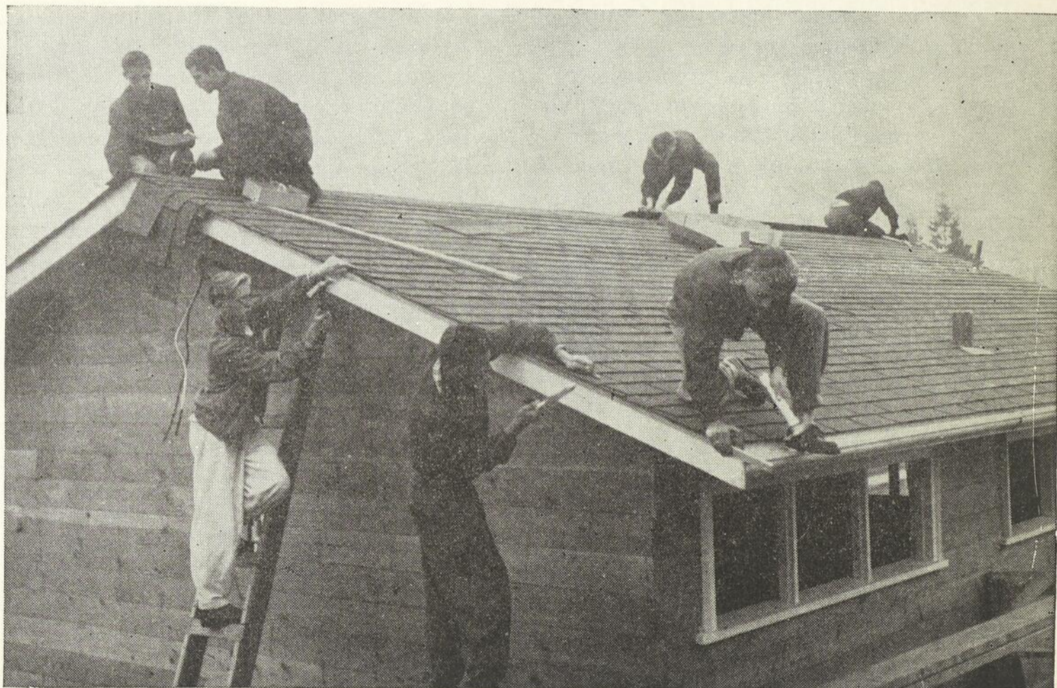
Boys learn all finishing operations to trim a roof properly.
