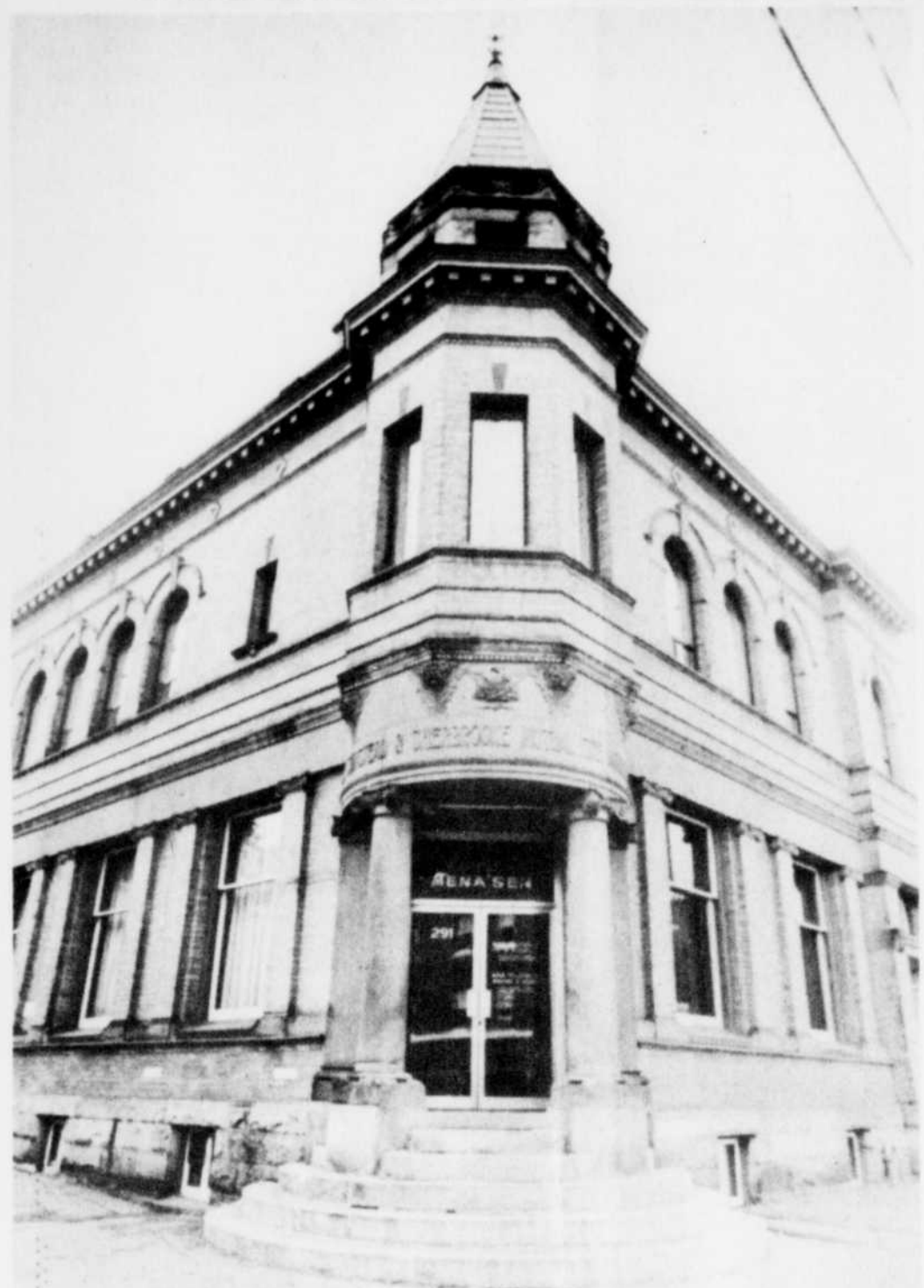
LANDMARK — The former offices of the Stanstead and Sherbrooke Insurance Company on Dufferin St., harken back to an era of dignified design in red sandstone. Although the original occupants have moved to their new offices on Prospect, it wasn't because the old headquarters were
