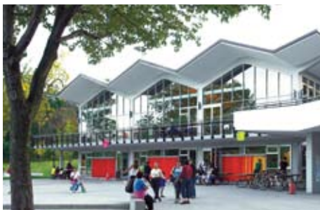
Beaver Lake pavilion after its restoration, summer 2006 © Ville de Montréal, Jean Landry.
