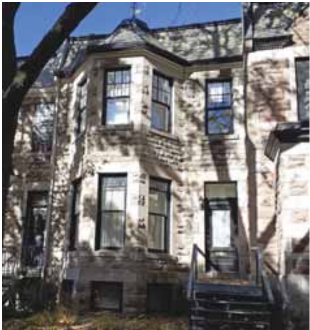
4477 de Maisonneuve, near Westmount Park, on October 26.
