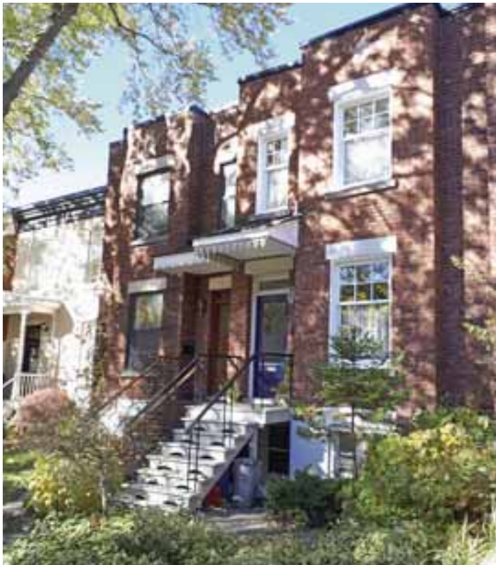
7 Ingleside, near Metcalfe and St. Catherine, on October 26.
