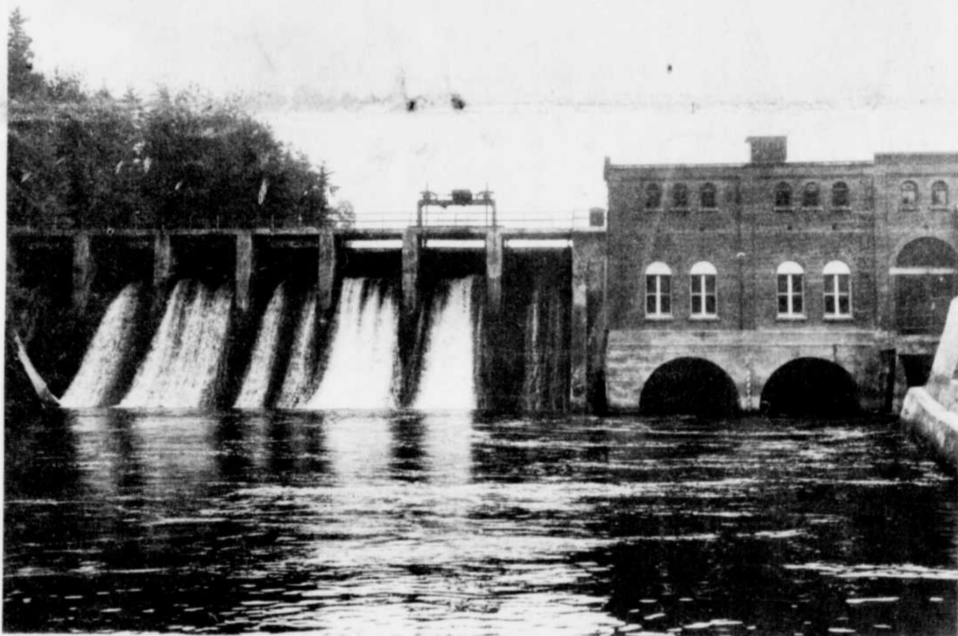
REAL POWERHOUSE — Built in 1911, the Rock Forest powerhouse provides close to 2,000 kilowatts for the
