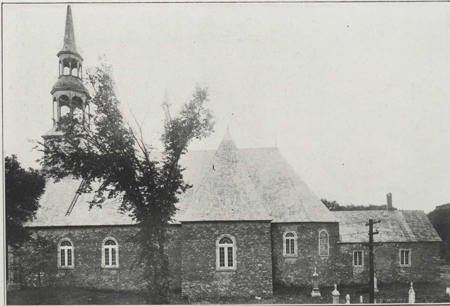
CHURCH OF VAUDREUIL: WEST SIDE
