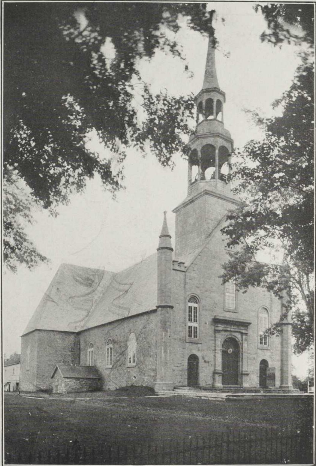
CHURCH OF VAUDREUIL: FRONT AND EAST SIDE
