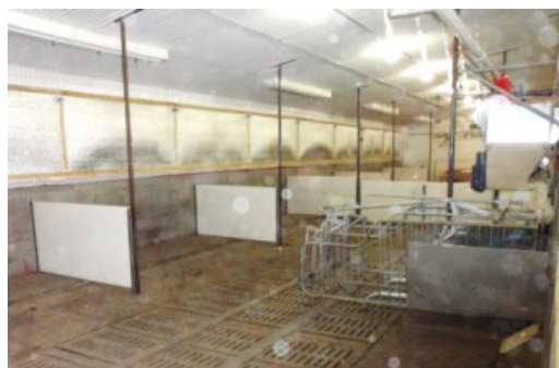
Figure 16 Equipment, PVC pen divisions and poles used to hold them securely
