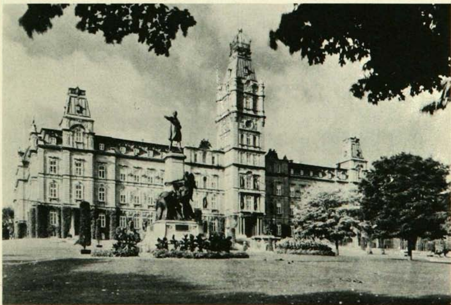
The Provincial Government Buildings, Québec
