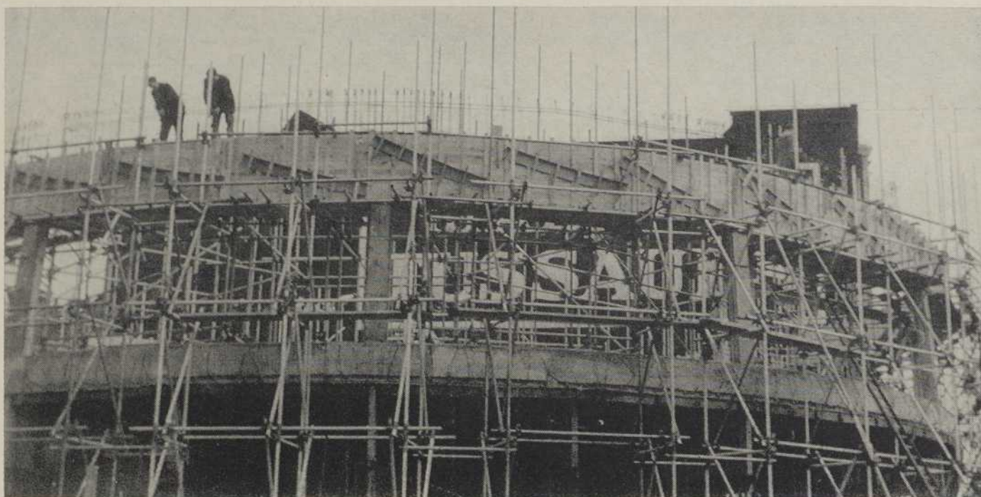
MADAME TUSSAUD'S PLANETARIUM DURING ERECTION
