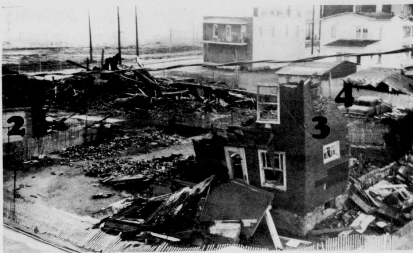
$150,000 FIRE DAMAGE — The burnt-out structures at the corner of Bourbeau Street and Penneton in Asbestos are shown here: 1. the Roberge block; 2. Au Rendez - Vous restaurant; 3. Bedard residence; 4. garages.
