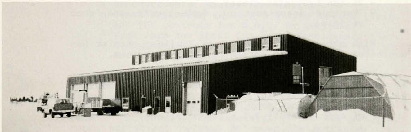
KIGIAK SERVICE CENTER IN KUUJJUAQ
