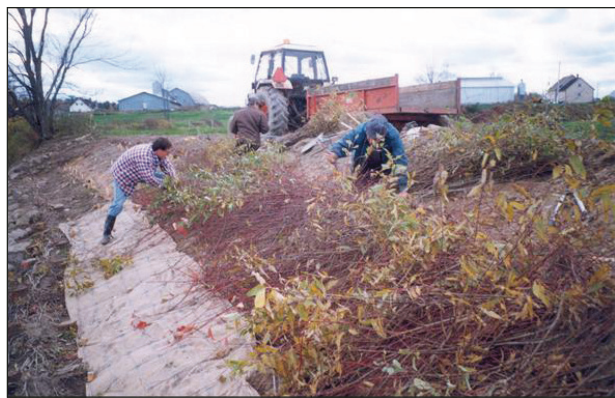
Photo 15: Installation de matelas de branches
