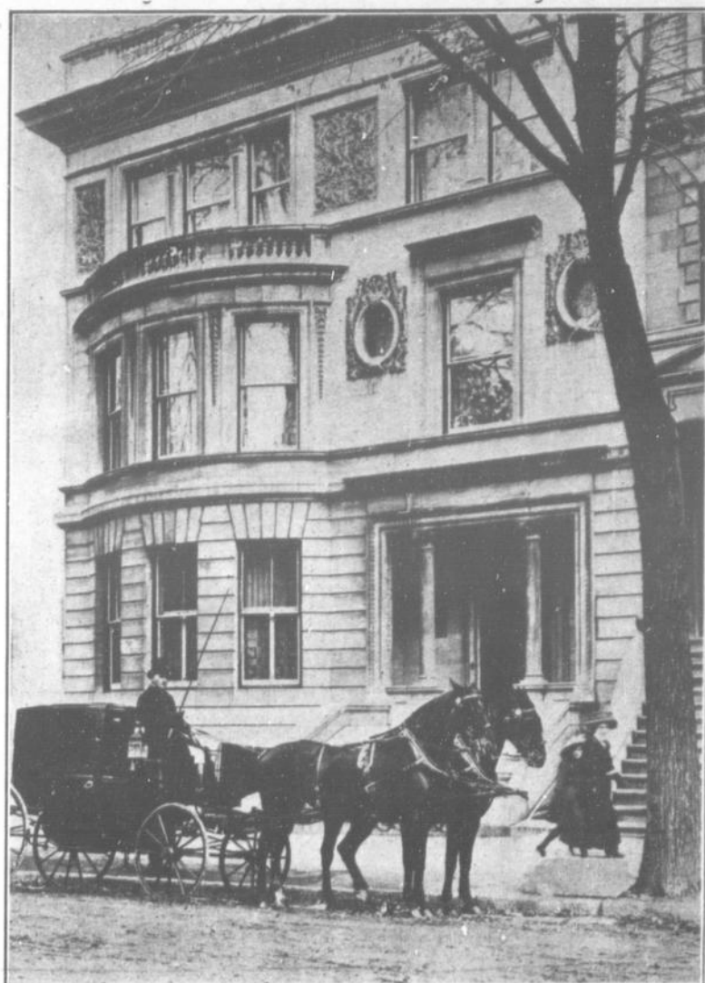
THE EXTERIOR IS OF STUDIED DESIGN AND CAREFUL EXECUTION.
