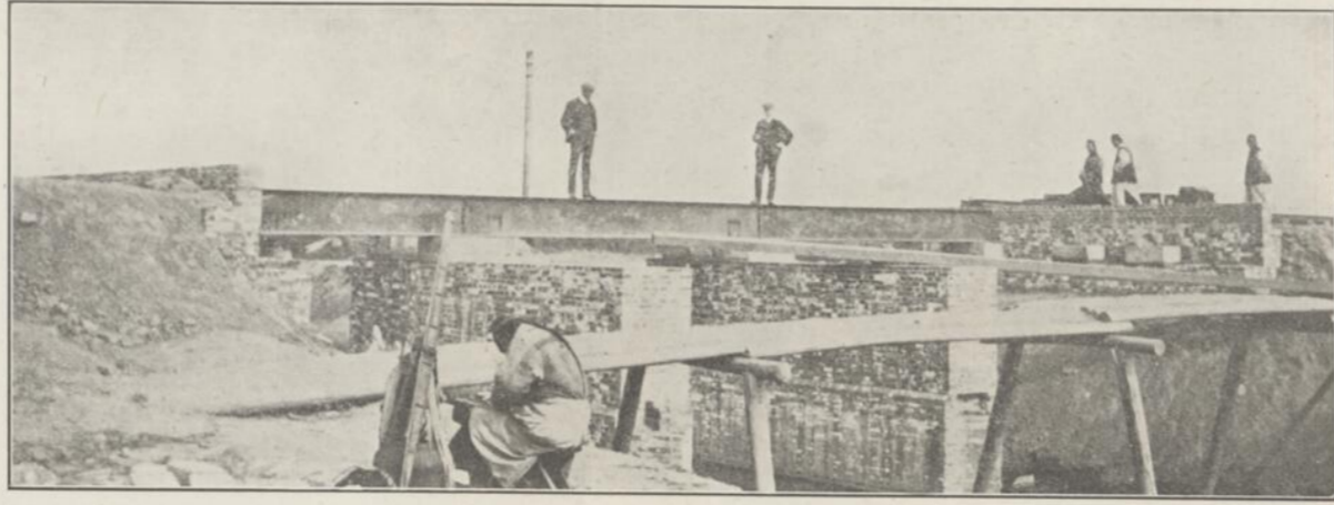
An incomplete railway bridge on the Shanghai-Nanking Railway.
