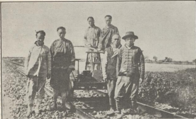
Survey coolies on the Shanghai-Nanking Railway, China, operating a hand-car. These coolies were of great assistance in constructing the road.
