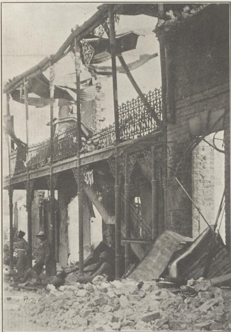
The Bank of Nova Scotia, Kingston, Jamaica, after the recent earthquake.
