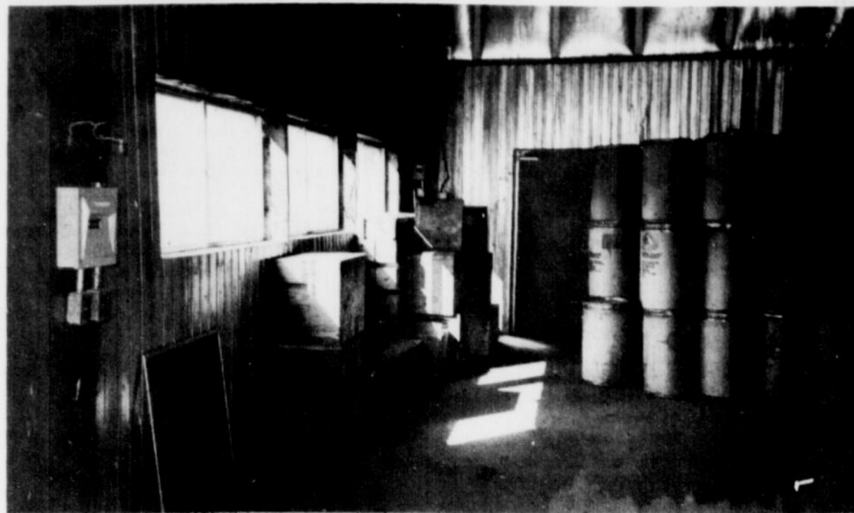
An inventory showed possible safety hazards remain in several buildings.
