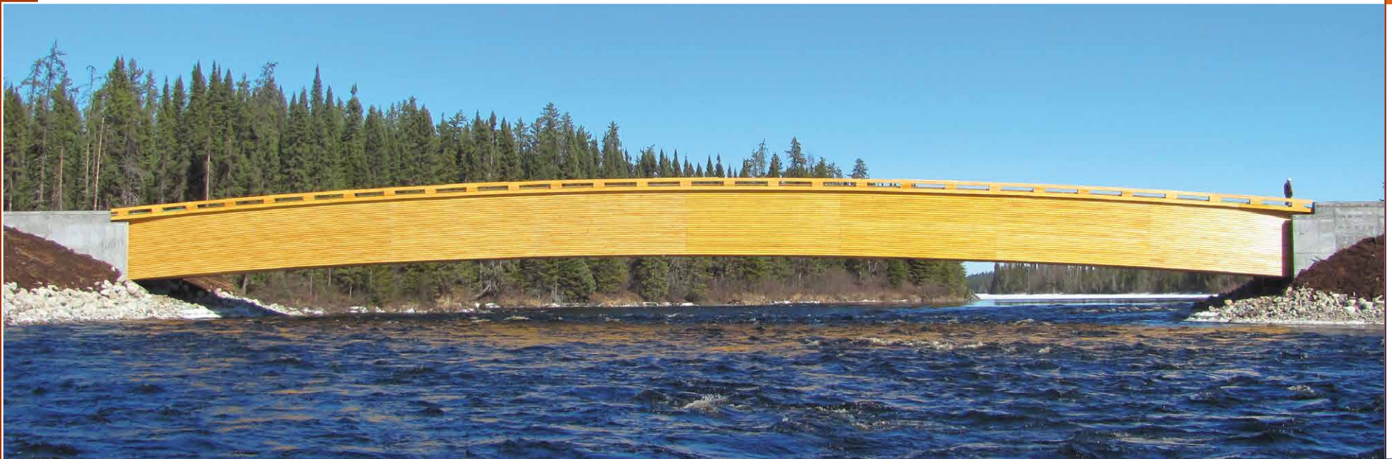
Maicasagi bridge Photo: Nordic Structures
