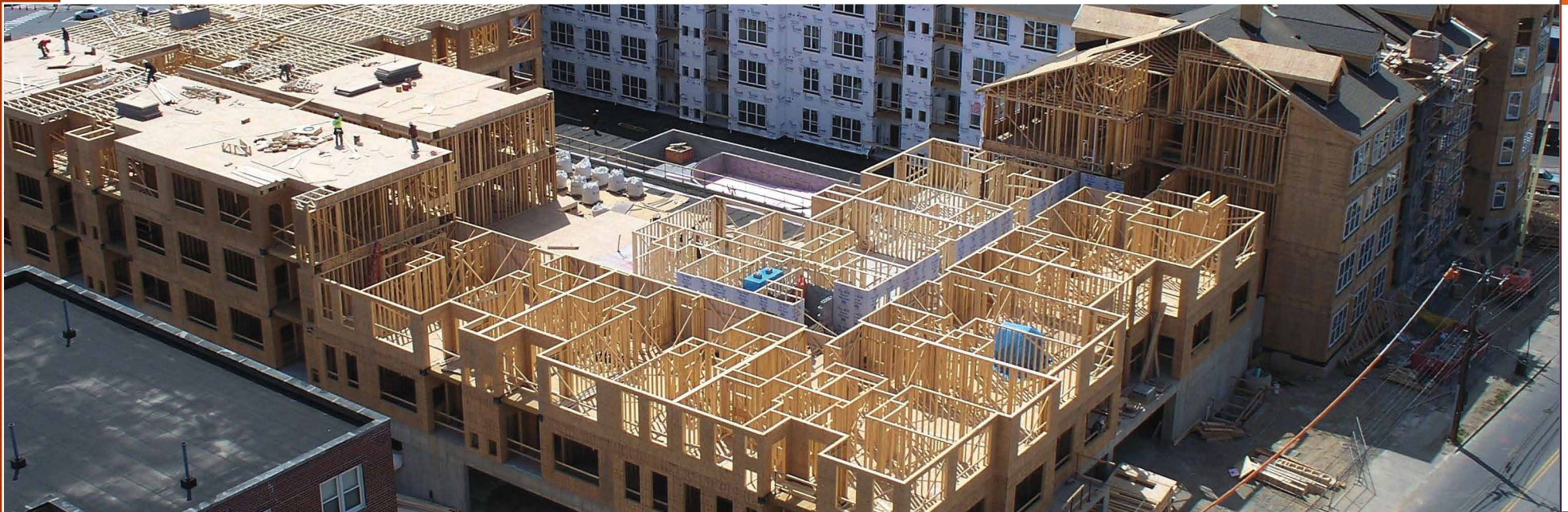
Multi-dwelling construction with a lightweight prefabricated frame Photo: Cecobois
