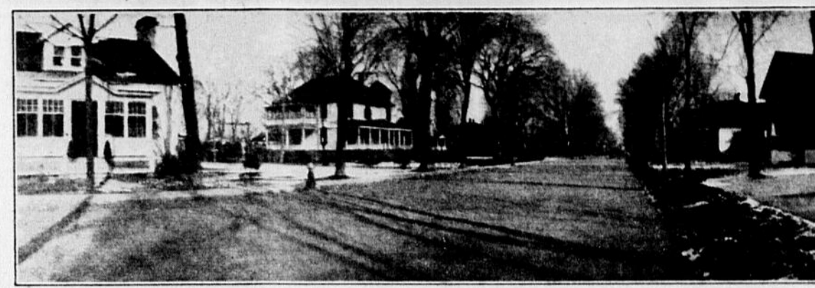
Huntingdon street called after Prince Arthur, now under construction as a Federal-Provincial unemployment relief scheme. This scene shows part of finished work. First home on left that of D. B. Kelly was eaten during Fenian Raids, and next home that of B. W. Allen was site of Presbyterian Church where ammunition and stores were kept.
