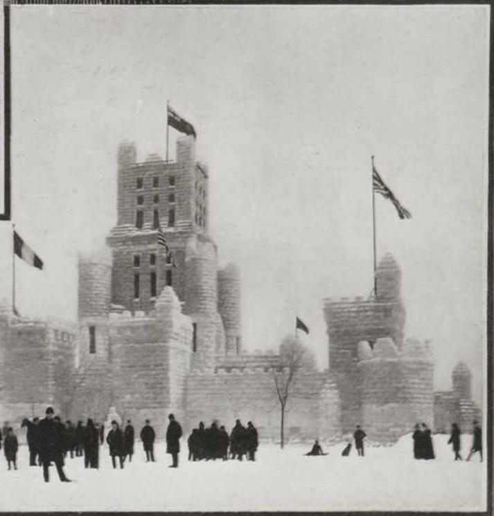
The Ice Palace. It is now about thirteen years since Montreal saw the last Ice Palace. It was built in Dominion Square on the spot where now stands the statue of Sir John A. Macdonald, and was in the form of an old castle, and built entirely of huge blocks of ice, which were from four to five feet long, and about two feet thick. At night time it was ablaze with electric lights and presented a most gorgeous and fascinating spectacle.
