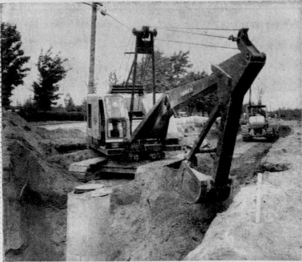
PIPE LAYING — A new sewer and water pipeline system is being installed in the northern section of Cowansville with the estimated cost being $190,000. The above photo is taken on Albert Street where the pipe laying excavation is taking place presently. Operating an earth remover is Rosaire Salois, a Cowansville worker.
