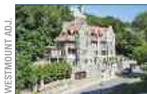
WESTMOUNT ADJ. 1210 REDPATH CRESCENT
