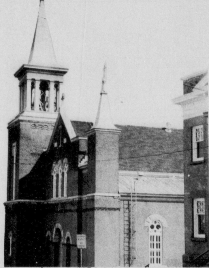
Cookshire's Catholic Church lost its steeple and tower
